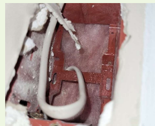
Wall insulation in some walls where renovated
