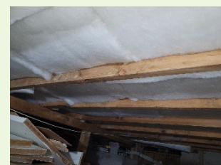
Space for infilling underfloor insulation with additional
